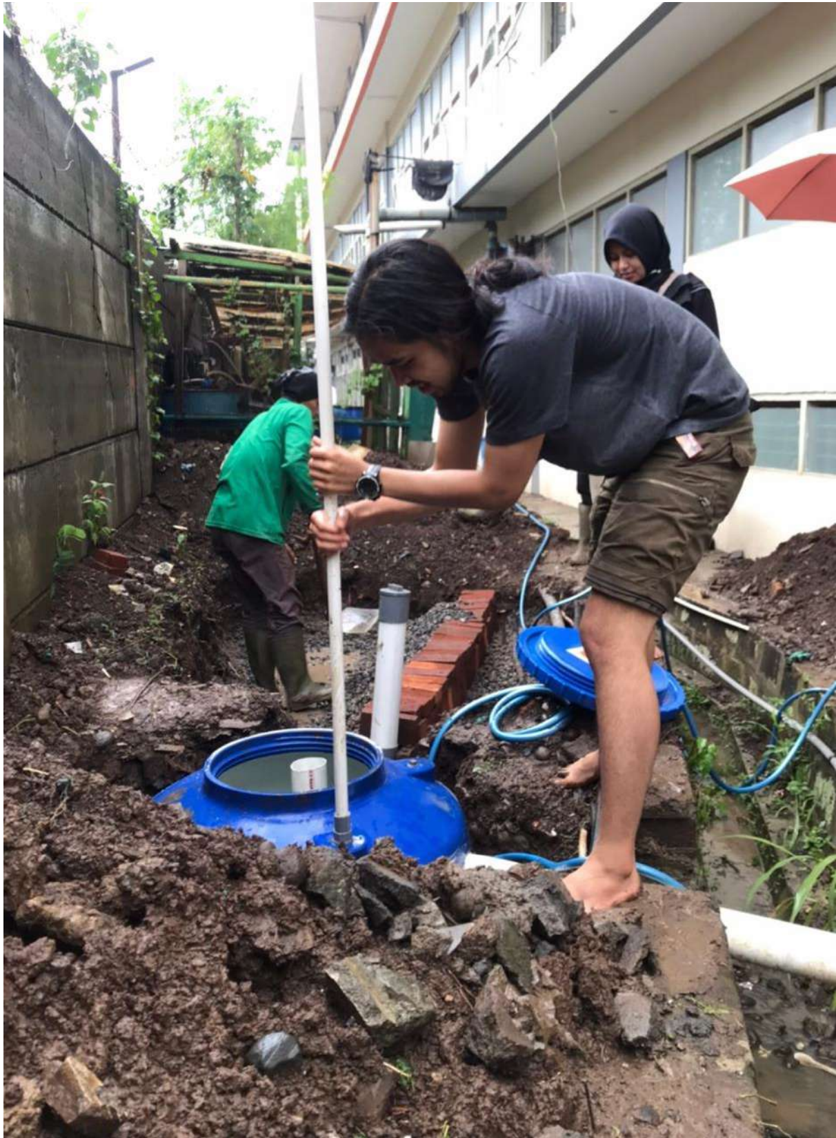
Figure 11.8 Installation of the tank and piping systems at Itenas site
