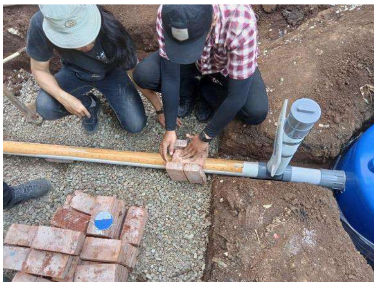
Figure 5.13 The Process of Installing Bricks Around Perforated Pipes
