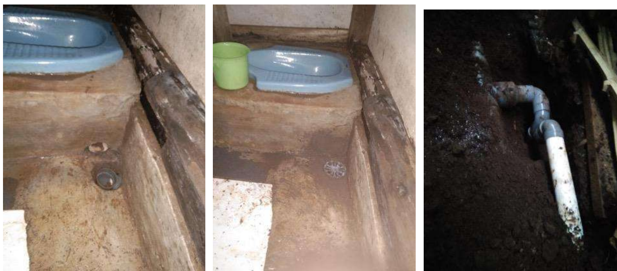
Figure 12.7 Wrongly constructed shower drain (before and after we fixed it) and newly installed p-traps
