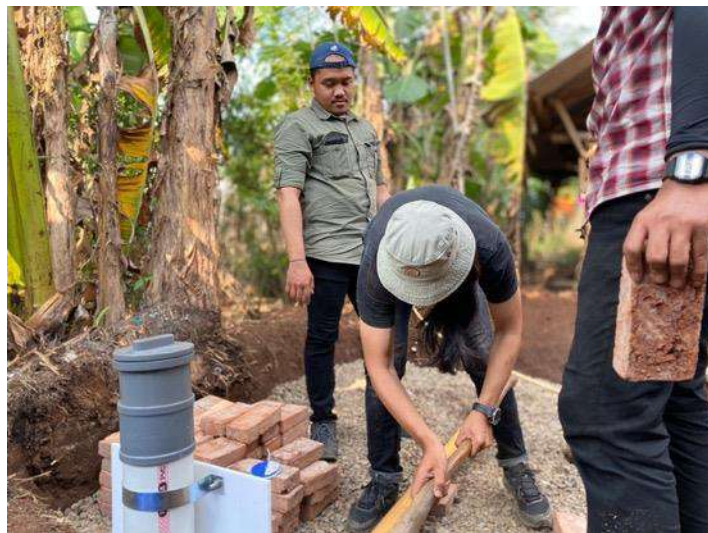
Figure 5.12 Process of distributing the Gravel at the bottom of the SWG garden
