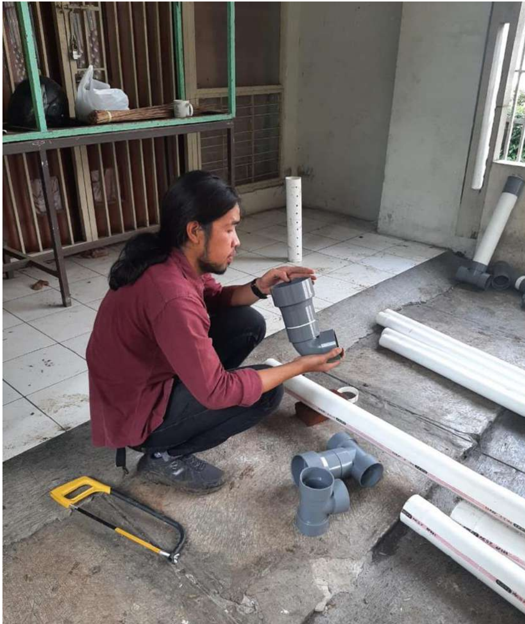
Figure 11.7 Preparation of piping systems for SWG at Itenas site
