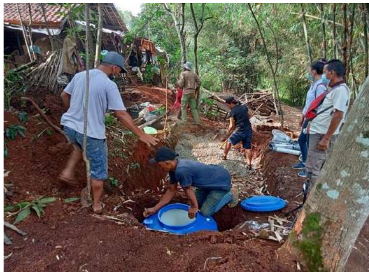
Figure 5.7 Local team and Team Install SWG Tank
