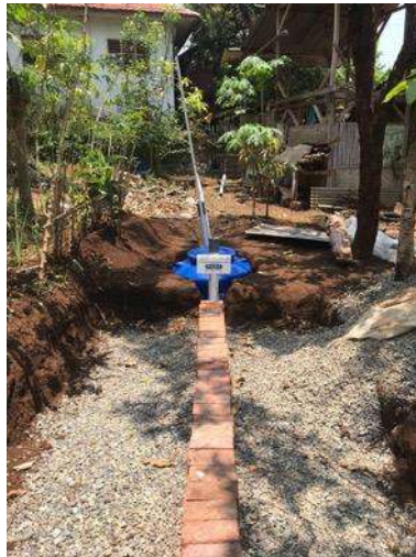
Figure 5.14 SWG Condition After Brick Installation
