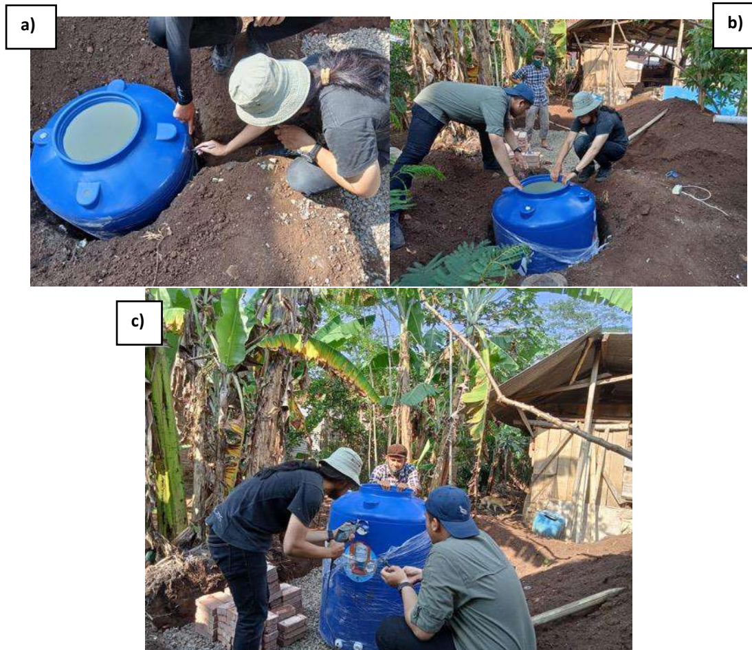
Figure 5.4 (a) The Process of Marking the Location of the Hole; (b) The process of making holes; (c) Tank Placement Process
