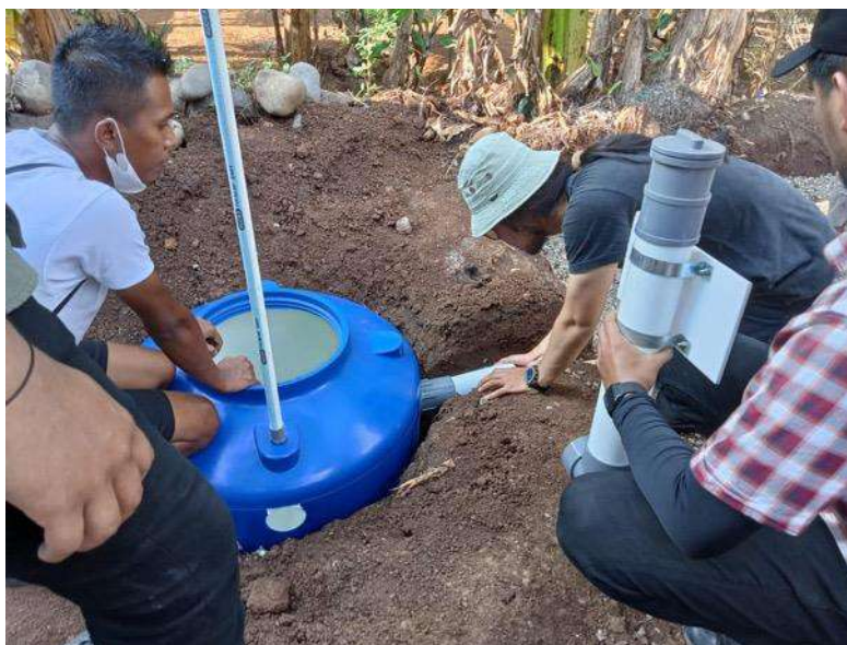
Figure 5.10 Connecting the pipes to the tank
