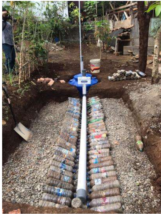
Figure 6.2 Example of SWB Installation in SWG Construction
