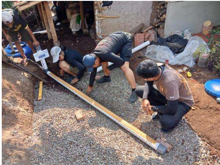
Figure 5.11 The Process of Installing Perforated Pipes from the Tank to the SWG Garden
