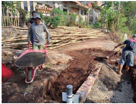
Figure 5.15 Process of adding sand (in between gravel and soil) by The Community and Team
