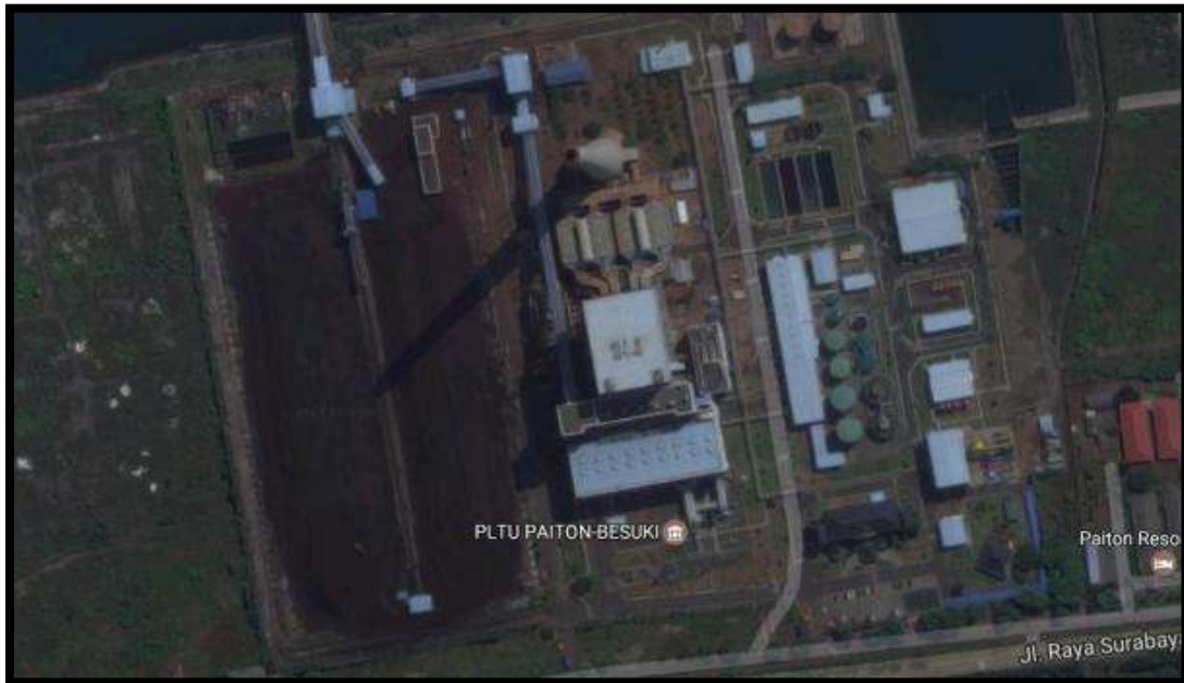
Gambar 2. Lokasi Survei Coal Yard PLTU Paiton
