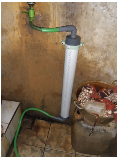
Gambar 7.6 Hasil Instalasi Alat Filter
