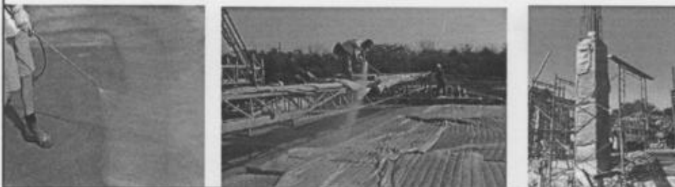
Schematic diagram of ideal curing of concrete by supplying water.
