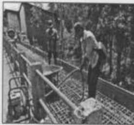
Fig. 7.11: Placing of poker vibrators (Based on ACI Manual of Concrete Practice.)
