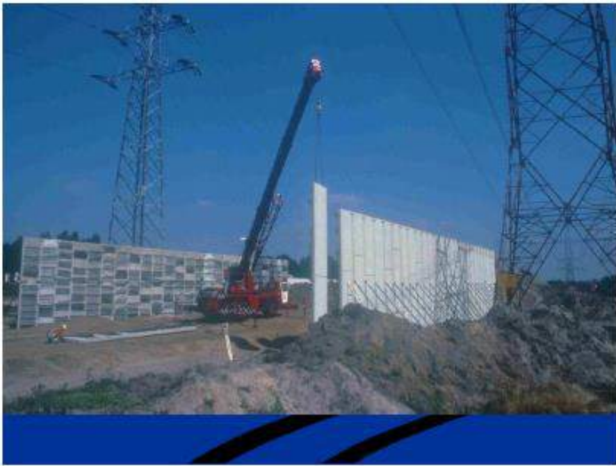
Full-height panel support to reinforced soil walls – rigid body rotation of facing
