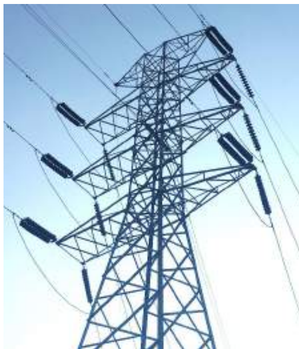
(e) Konfigurasi ST / DT ( Suspension Disc )
