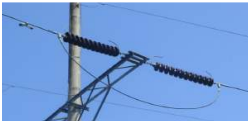
(c) Konfigurasi ST/ST ( Suspension Disc )
