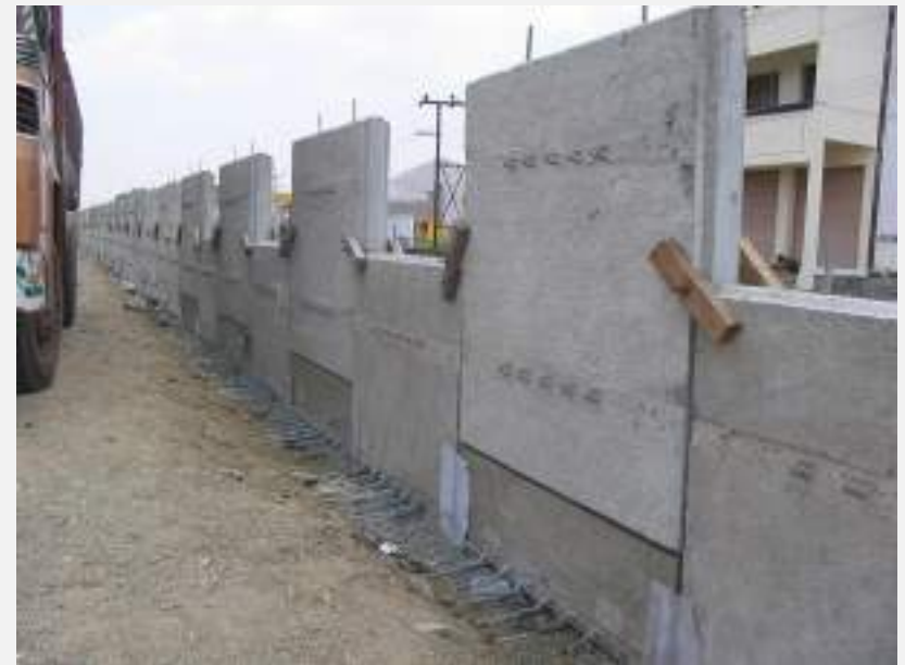
Incremental panel support to reinforced soil walls – bulging type deformation at front end
