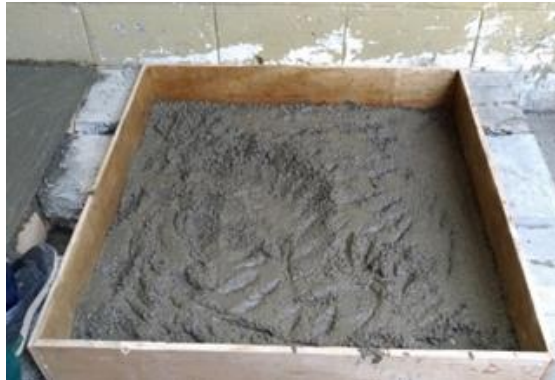
Gambar 6. Proses pengisian lapisan kulit pelat floating concrete
